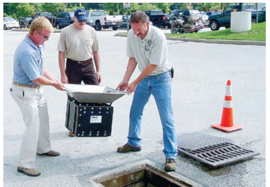
Bob Kelly, City Engineer; Chris Stuhm, Facilities Manager; and John Biro, Westlake Service Department Fabricator install a catch basin insert. Photo by Jim DeVore
